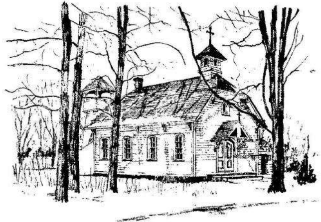
ST. BARTHOLOMEW'S CHURCH ABOUT 1914
